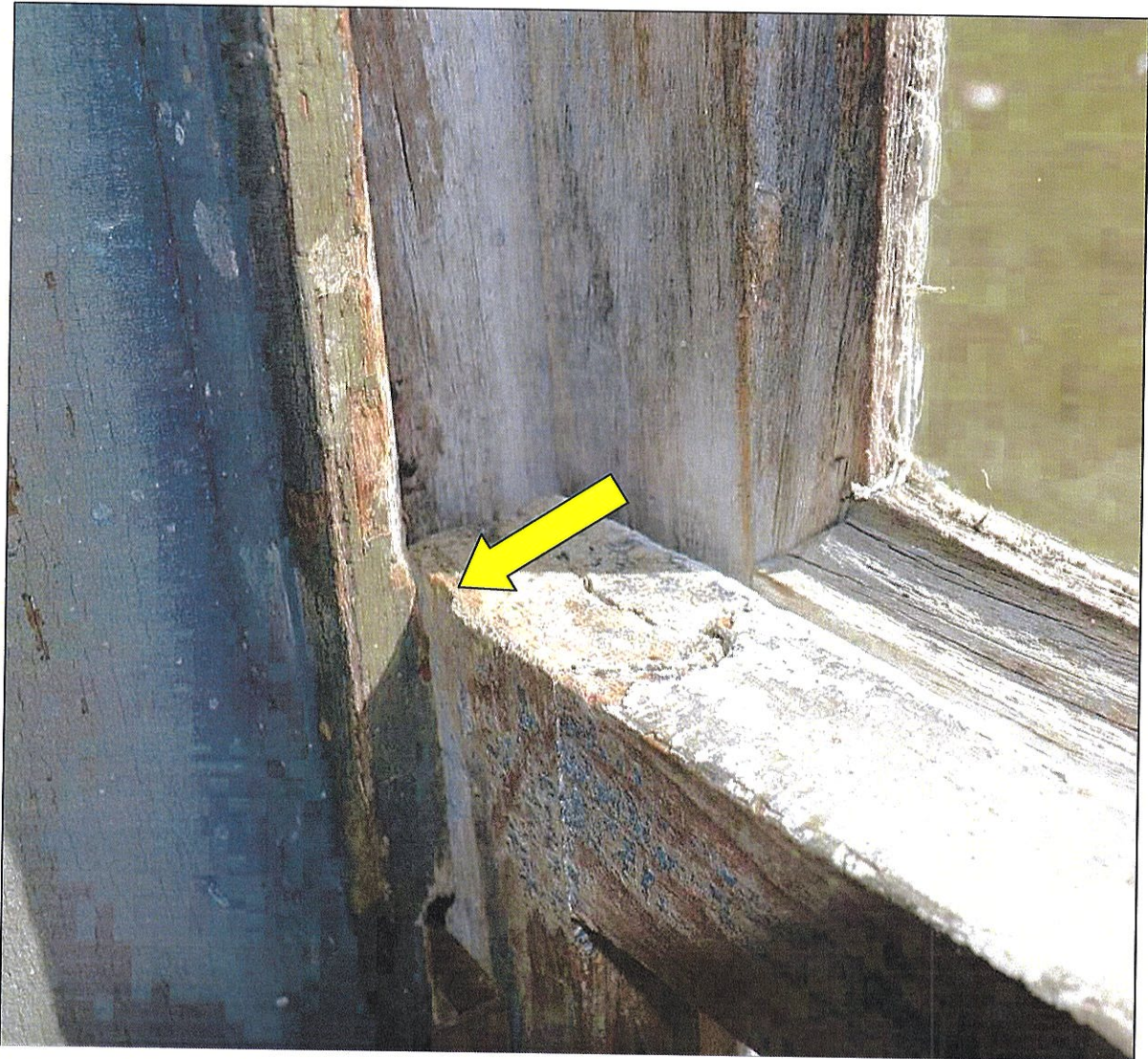
Detail of the meeting rail of a lower sash on the south end of the third floor, as seen in the right-hand drawing on the preceding page. The shallow rabbet in the stile does not match the width of the existing window stop. Other windows on this floor should be examined for further evidence of original window stops or of possible other explanations of the shallow rabbet.
