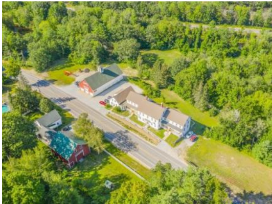
Route 103, Warner, NH, A 19th Century farm on 2 acres converted to eleven residential units
